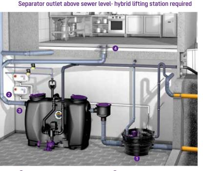
Properly sized hybrid lifting station
